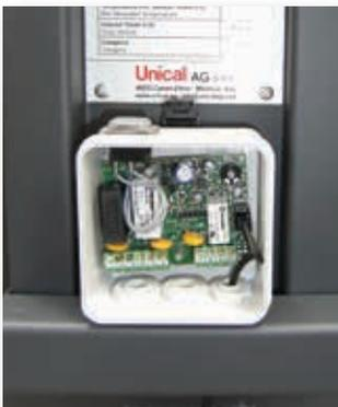
■ Temperature regulation system, with NTC sensor
